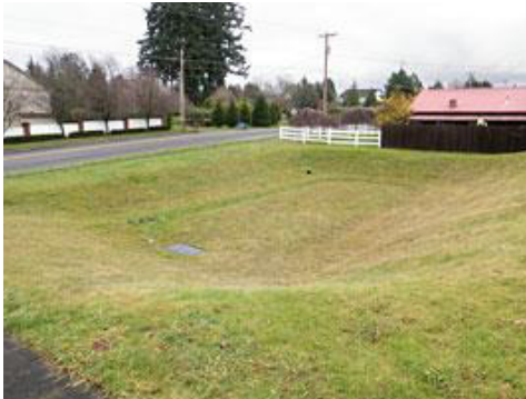
Figure 41. Small grass stormwater basin infiltrates runoff
